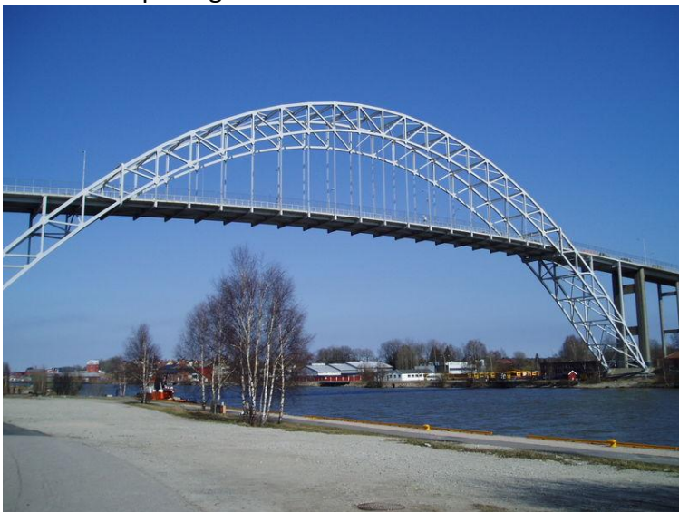
Bridge of Fredrikstad
